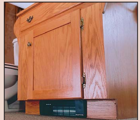
Twin-Flo III heater bathroom cabinet installation.
